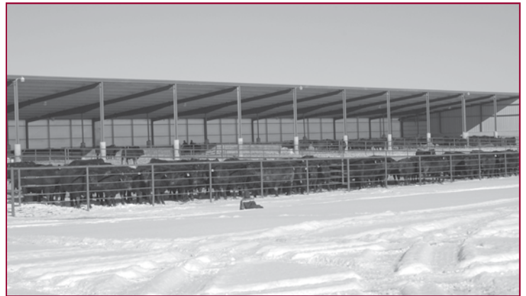
Our State-of-the-art sale facility in Kimball, MN
